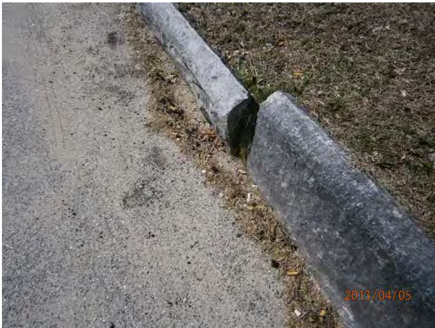
3. Stone retaining wall - curb leaning
