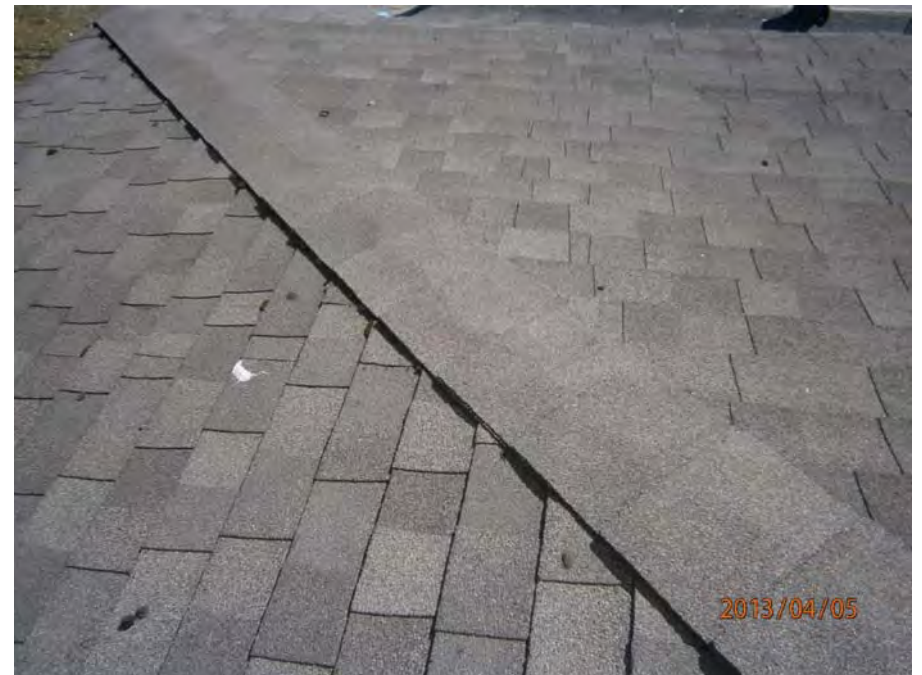
12. Architectural grade roof shingles
