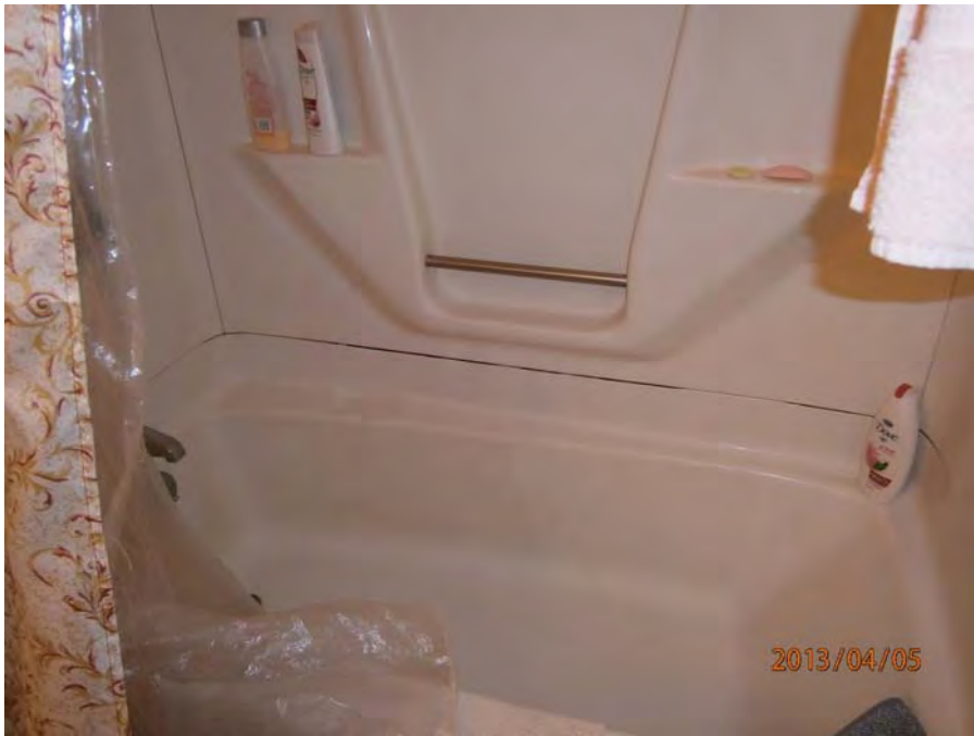
21. Unit fiberglass tub and walls
