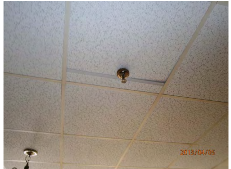
24. Unit ceiling tile and sprinkler head
