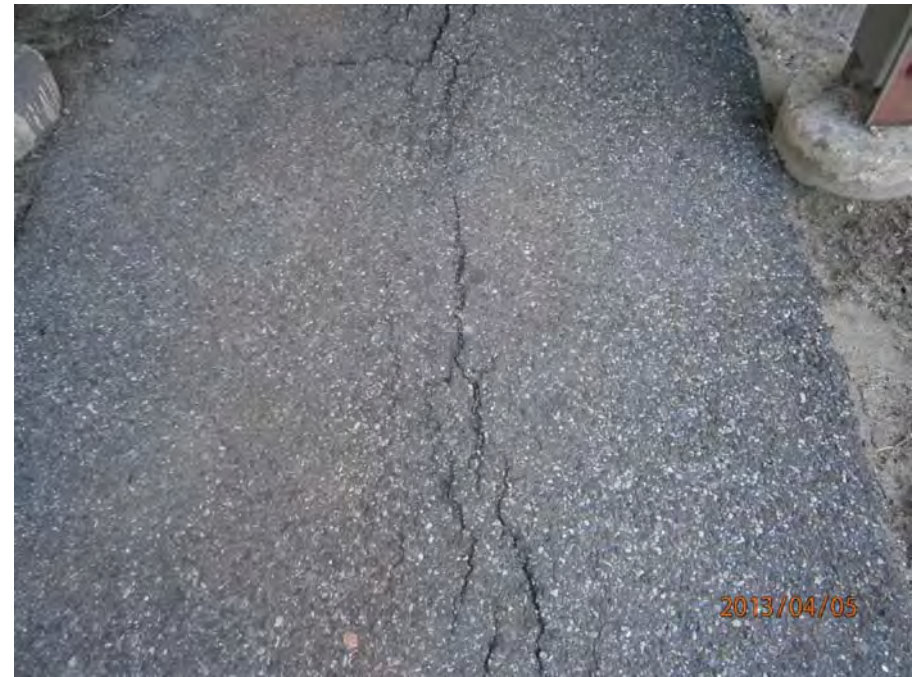
2. Asphalt walkway - minor cracks
