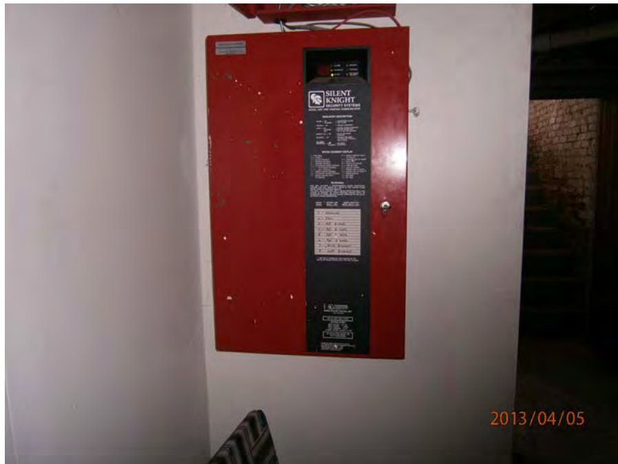
15. Zoned fire control panel
